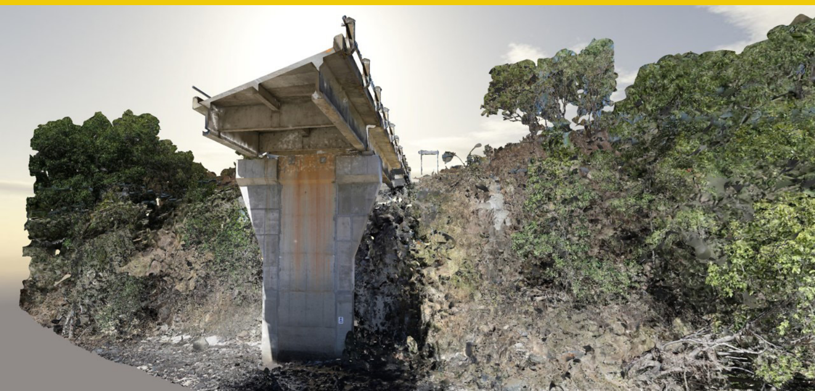
Image above - preparation of the reality model in Context Capture - thousands of images, survey control and laser scan together. Image below - Survey-grade reality mesh as a result from above model post-processing.
